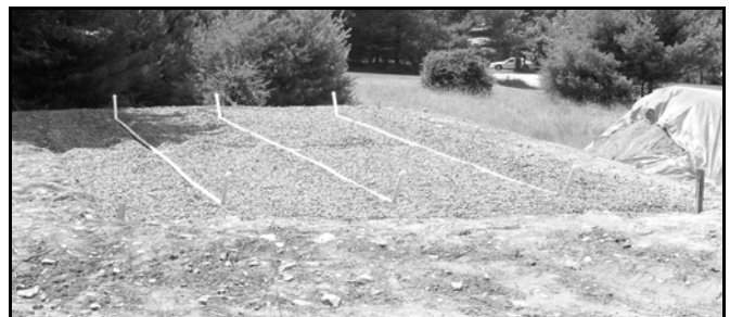
Sand Mound Under Construction
